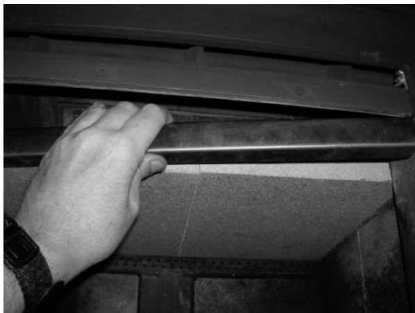
Figure 19a – Removing / Replacing the Baffle
